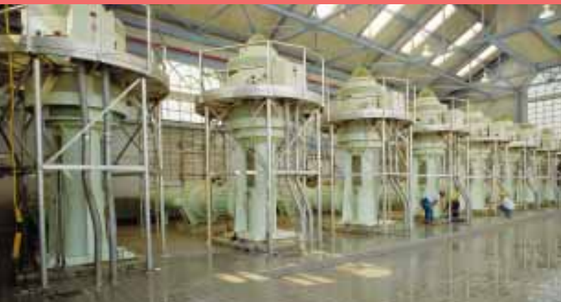
Ingersoll-Dresser Pump Company's expertise in the water resources industry is applied at the Hemphill Pumping Station in Atlanta, where eight vertical turbine pumps help meet the city's water supply needs.
