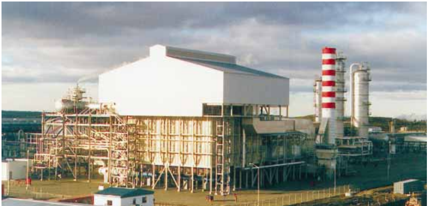
The Methanex facility in Puntas Arenas Chile is the largest methanol producing complex in the world.
